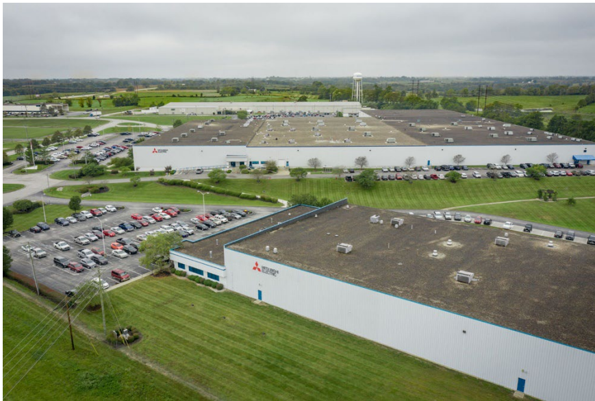
Exterior of the planned U.S. manufacturing site
