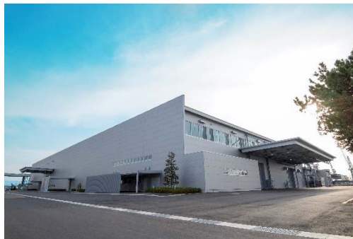
New integrated-automation vacuum interrupter and circuit breaker factory
