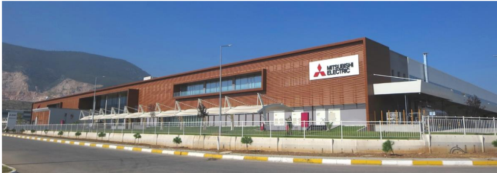
مصنع Mitsubishi Electric Air Conditioning Systems Manufacturing Turkey (المصنع ١)
