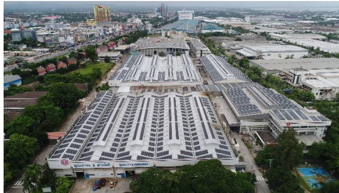
Siam Compressor Industry Co., Ltd
